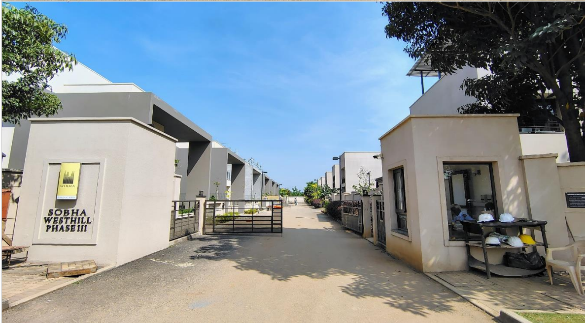
Sobha West Hill Part C Coimbatore
