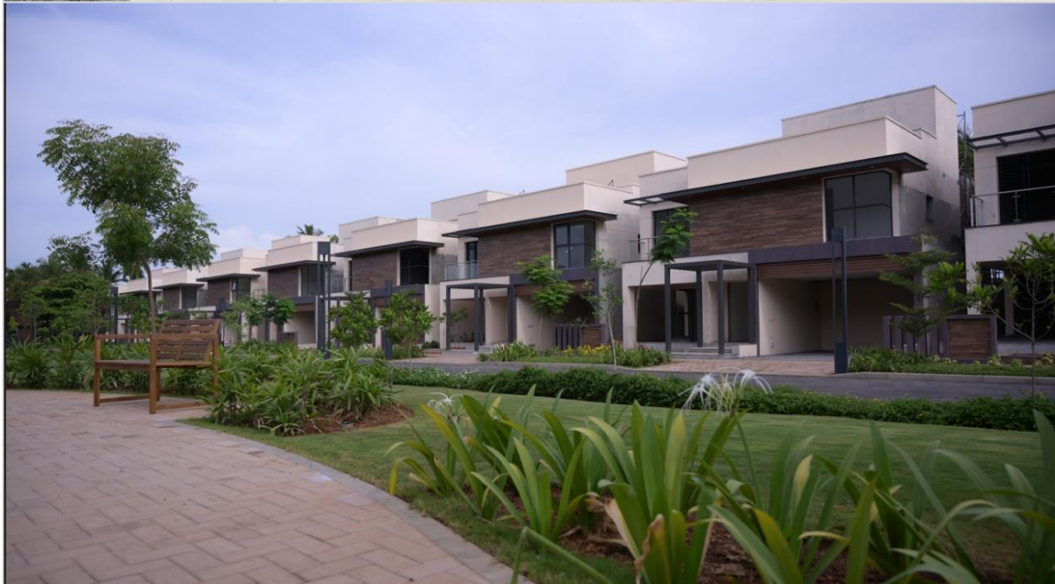
Sobha Silver Estate Thrissur
