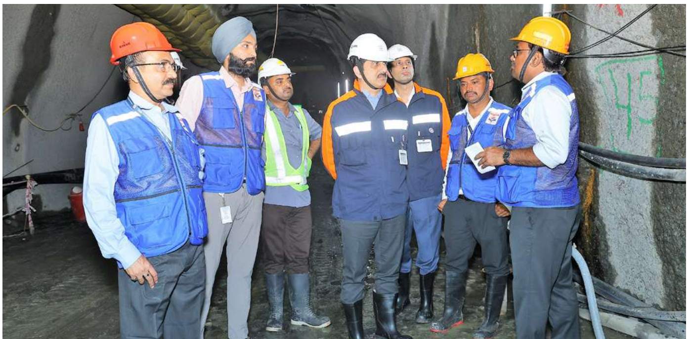
Visit of Director-HR to Mangalore LPG Cavern Project
