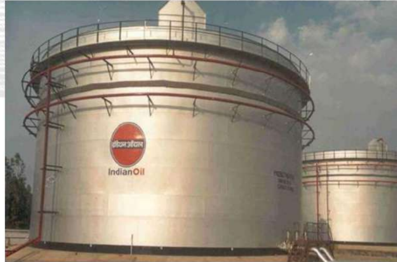
Cone / Dome Roof Tanks
