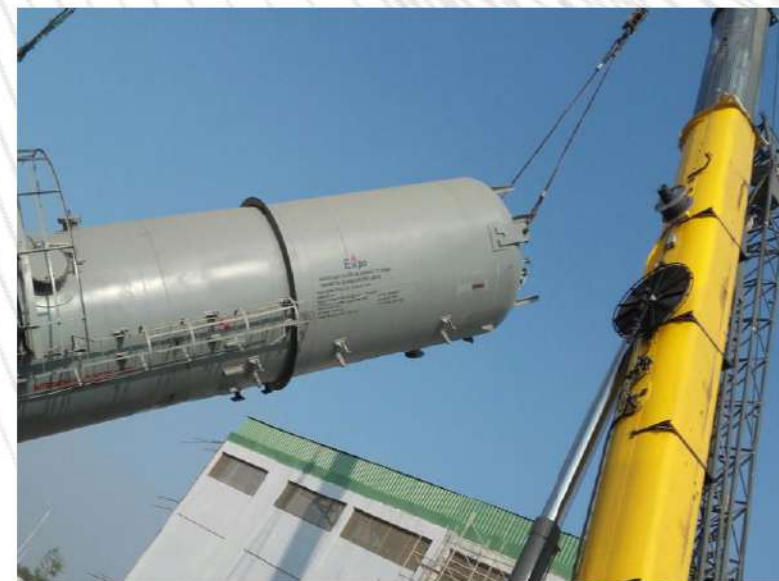
Fabrication & Erection of Equipments
