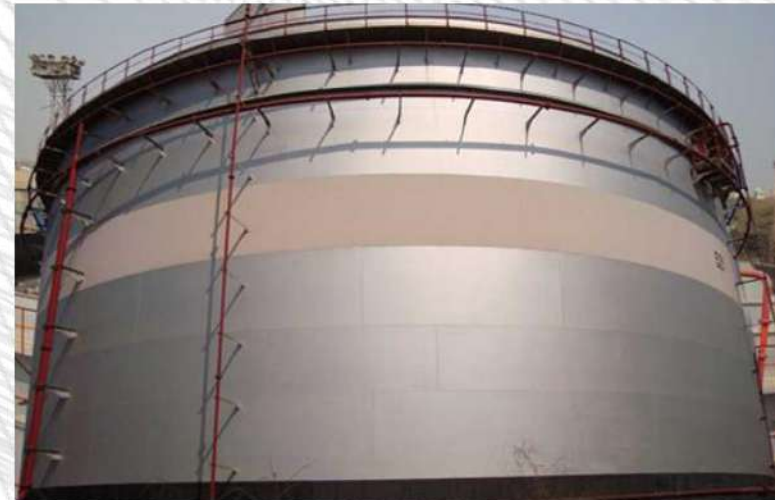
Floating Roof Tanks
