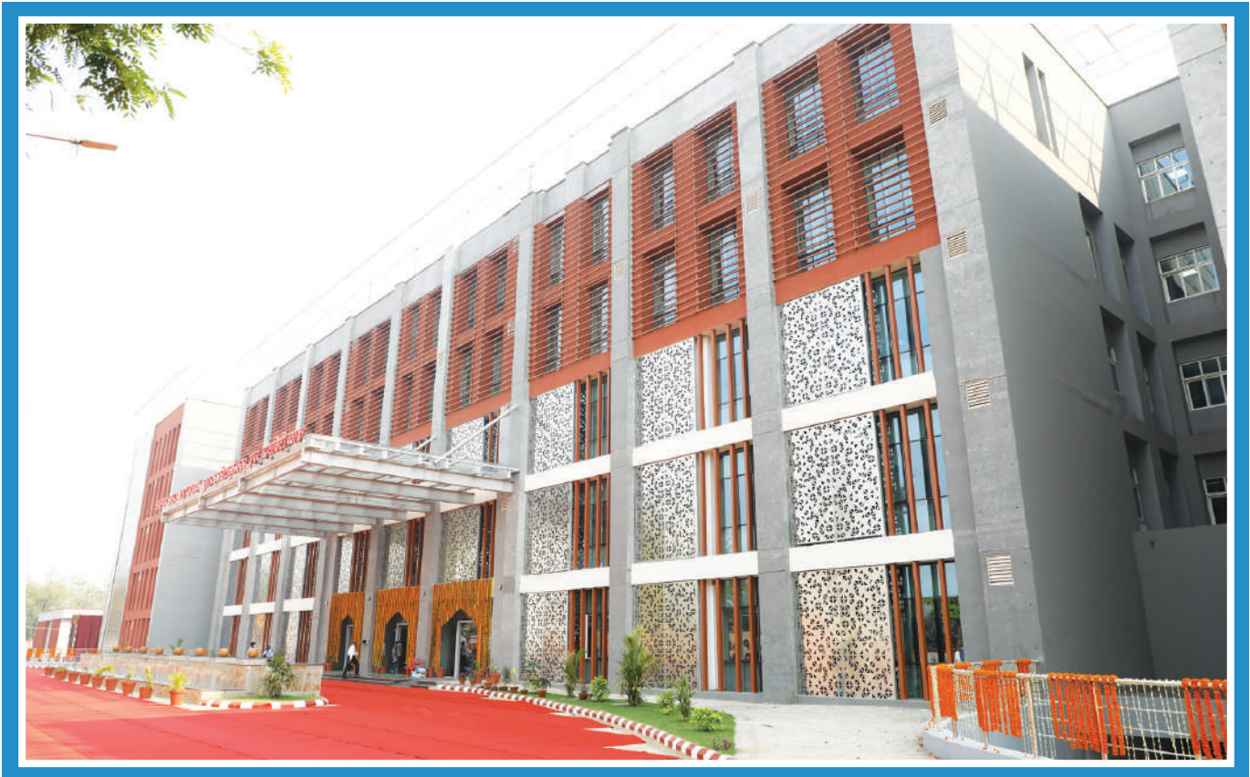
Super Speciality Hospital, Rourkela, Odisha
