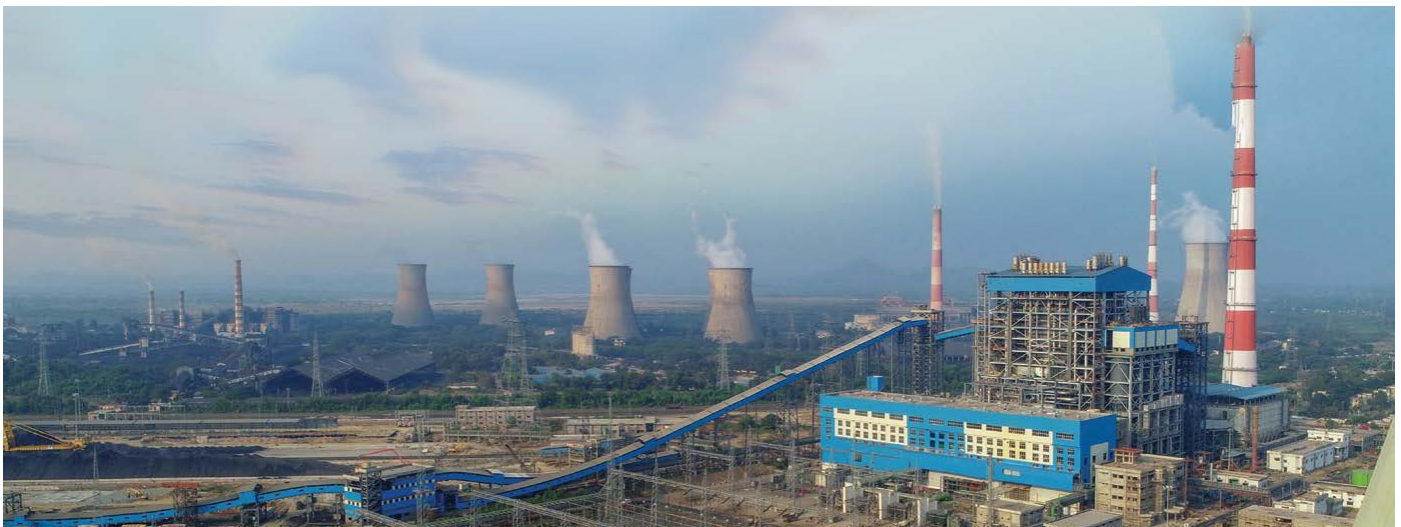
Kothagudem Unit 12 (800MW) commissioned by BHEL, achieved highest PLF of 85.5% and OA of 94.4%, among BHEL supplied supercritical sets
