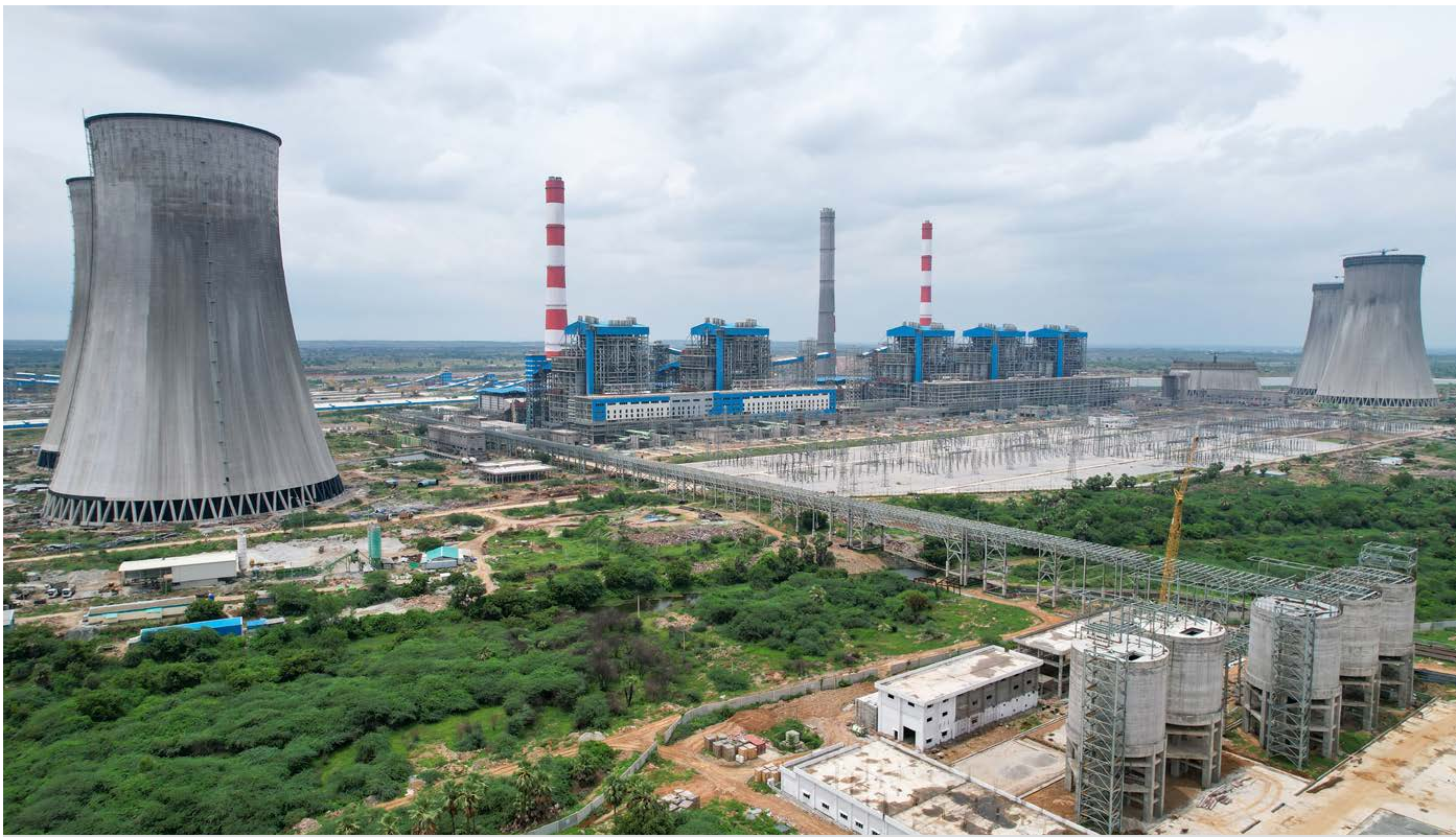
BHEL has manufactured India's first set of catalysts for Selective Catalytic Reduction for limiting NOx emissions for the 5x800 MW Yadri Thermal Power Station in Telangana
