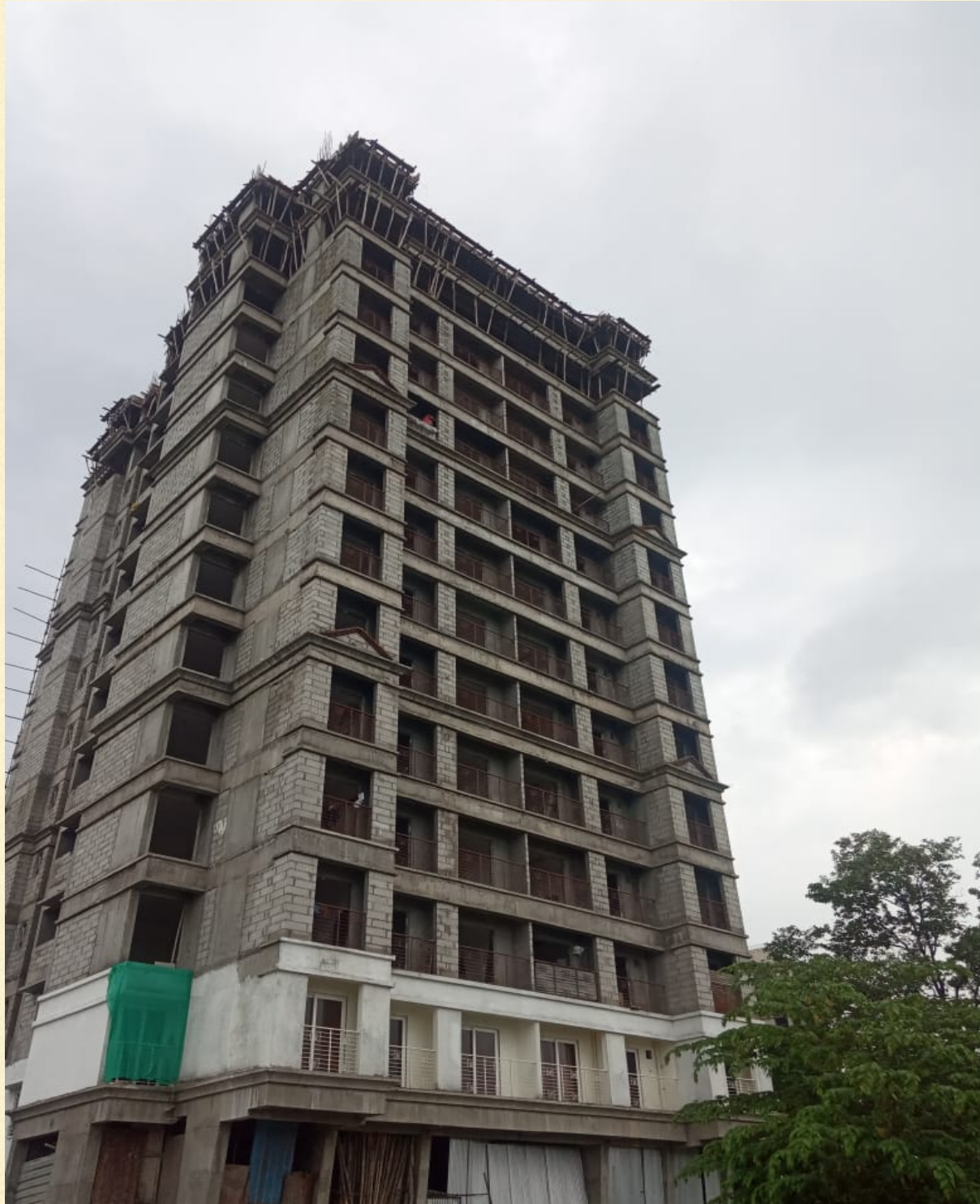
14 th floor completed
