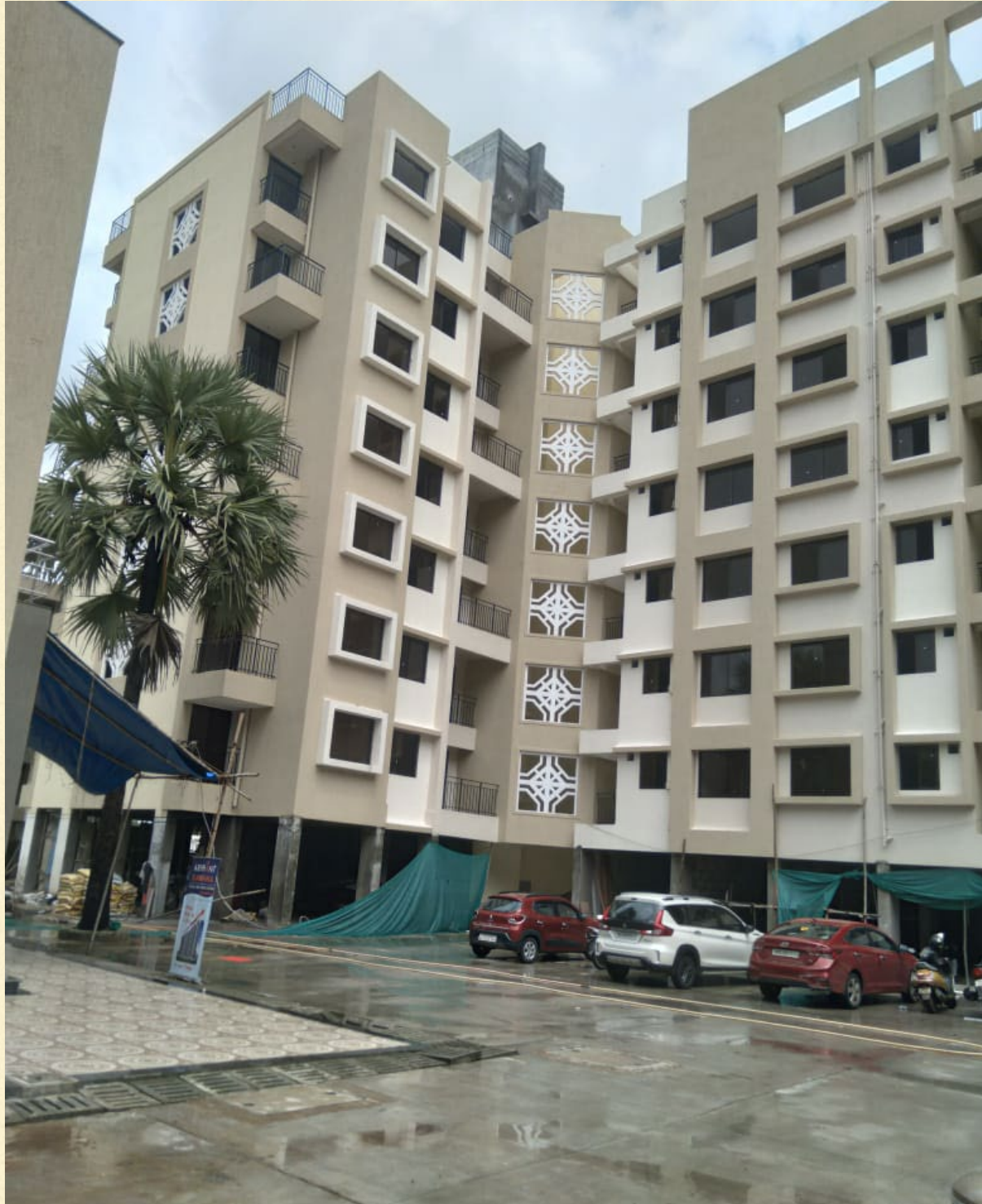
Internal finishing in progress
