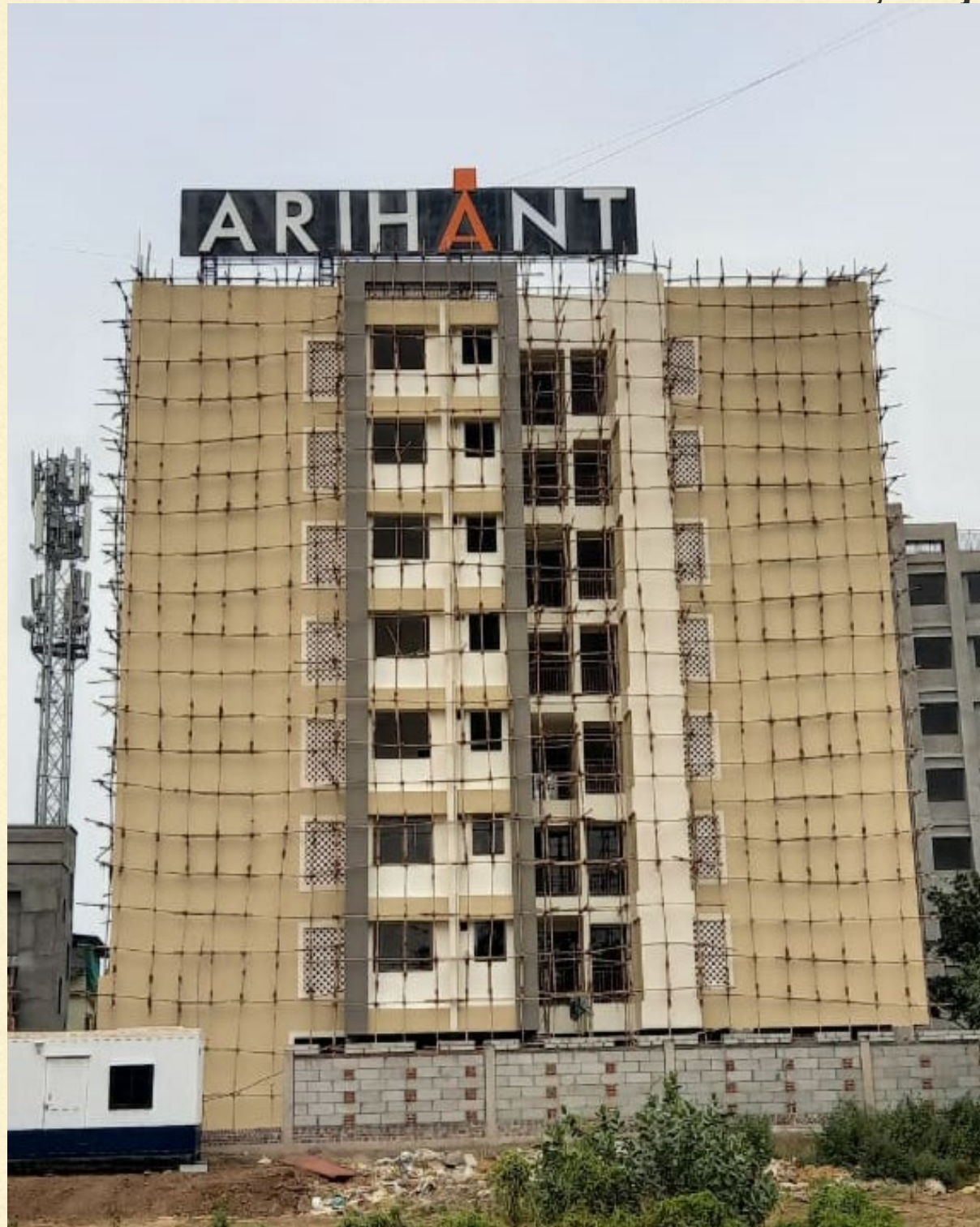
Painting, flooring, firefighting works in progress
