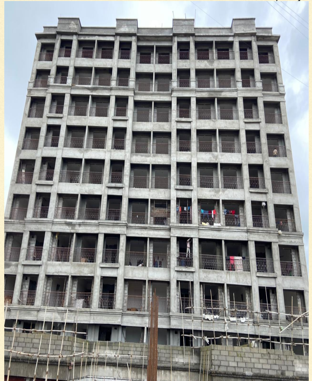
Internal finishing work in progress in Wing-B2
