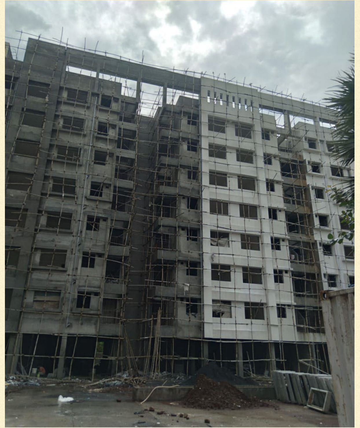
External painting and finishing in progress
