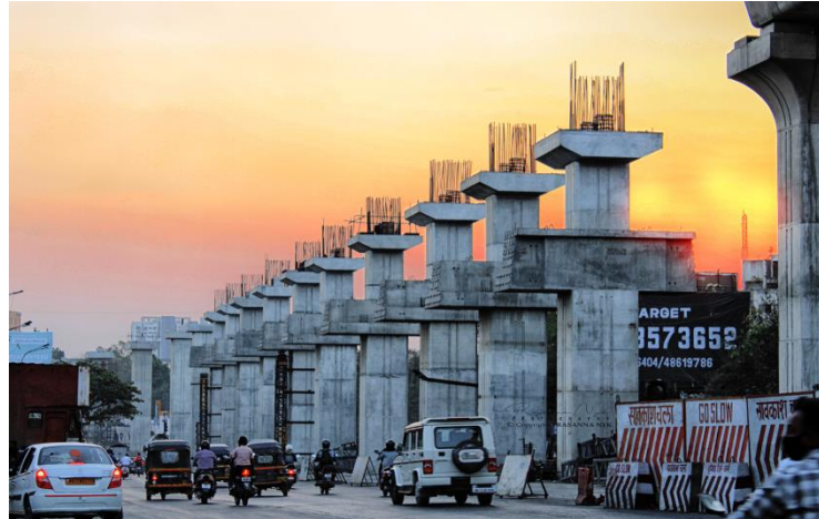
Pune Elevated Metro
