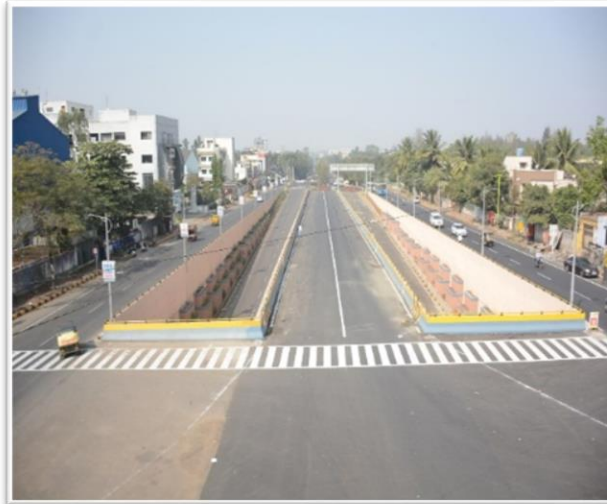
KSB Underpass, Pune
