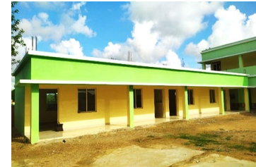
Construction of 2 classrooms at local school in Balasore
