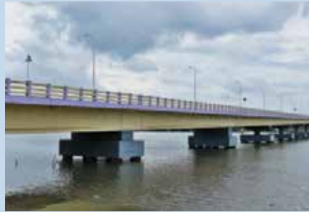
Thevara Bridge (Kerala)
