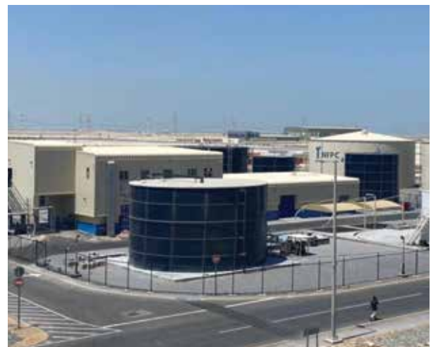
||||| NFPC Effluent Treatment Plant, Abu Dhabi
