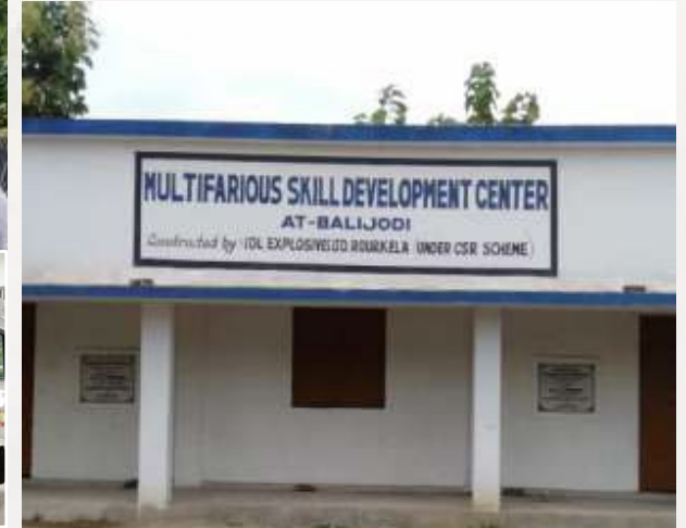
Multifarious Skill Development Center built under CSR at Balijodi, Orissa
