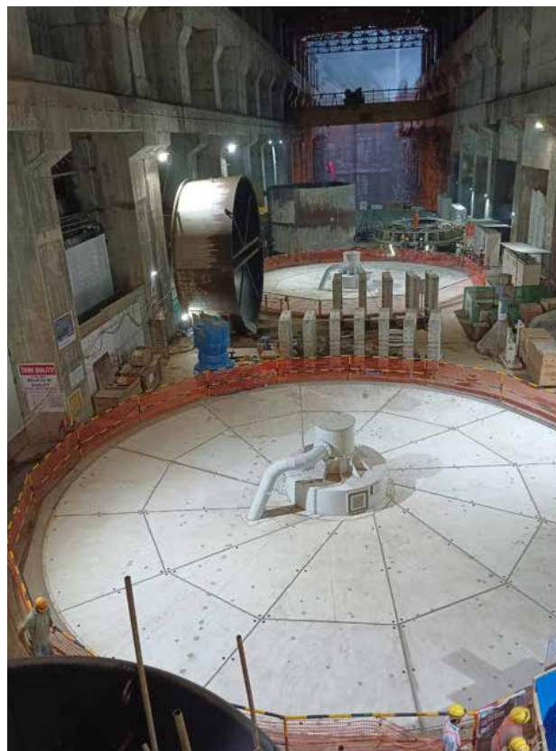
BOXING UP OF UNIT#1 & UNIT#2 (250 MW EACH) COMPLETED – 2000 MW SUBANSIRI LOWER (ARUNACHAL PRADESH)
