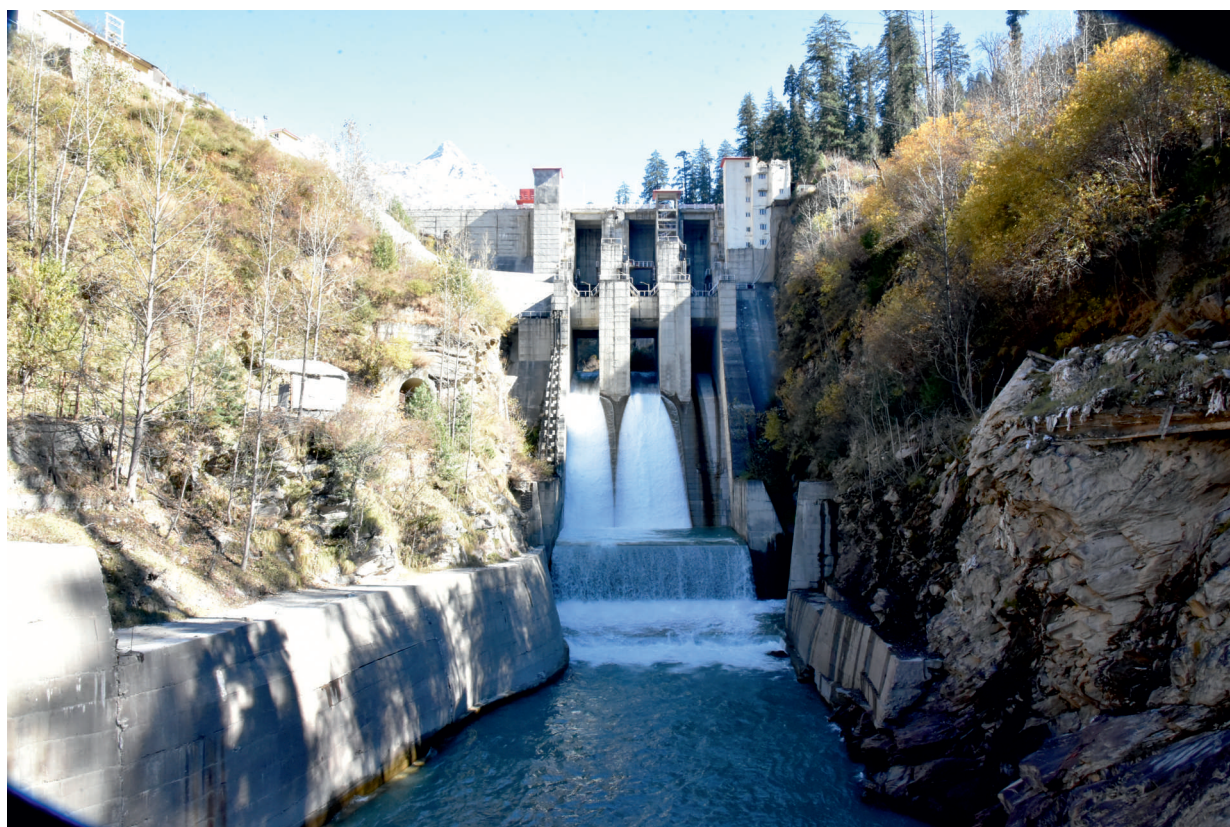
800 MW Parbati-II Project (Himachal Pradesh) – Dam
