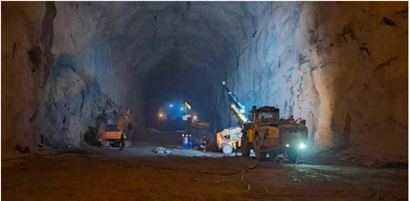
POWER HOUSE CAVERN EXCAVATION- 850 MW RATLE (UT OF J&K)
