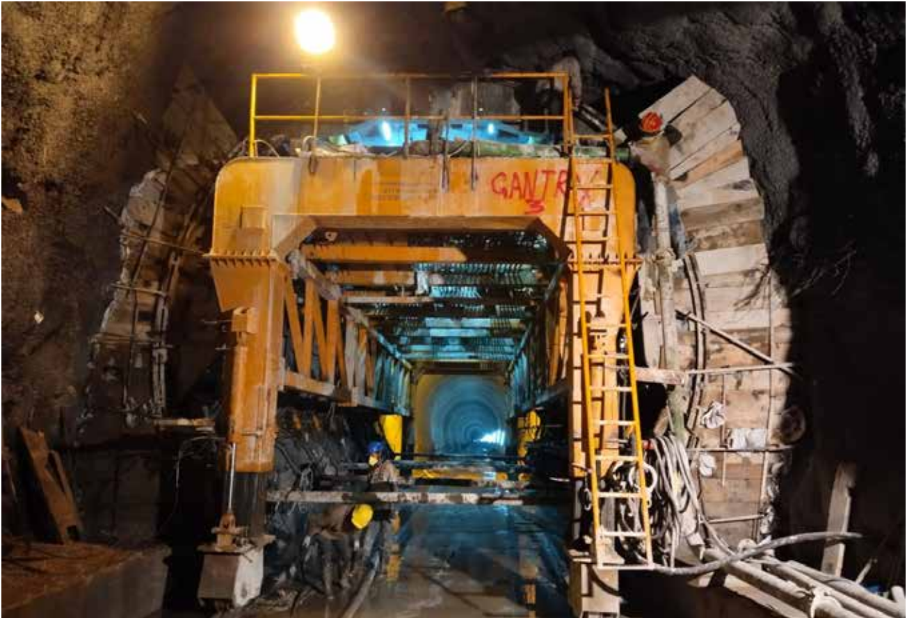
LINING WORKS IN FACE-3 & FACE-4 OF HEAD RACE TUNNEL – 800 MW PARBATI-II (HIMACHAL PRADESH)
