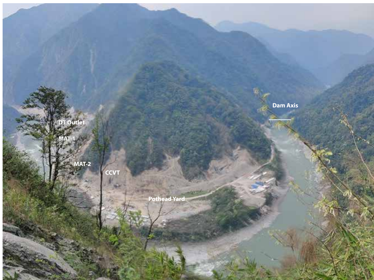
PANORAMIC VIEW – SITE OF 2880 MW DIBANG MULTIPURPOSE PROJECT (ARUNACHAL PRADESH)
