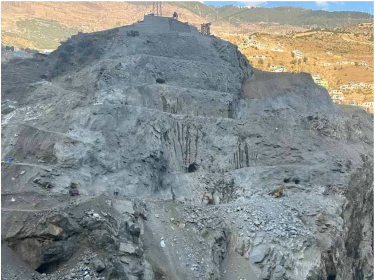
DAM ABUTMENT STRPPING- 850 MW RATLE (UT OF J&K)
