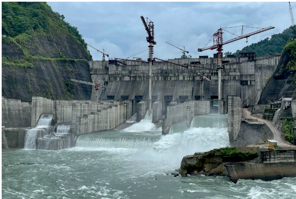
2000 MW Subansiri Lower Project (Assam/Arunachal Pradesh) - Dam
