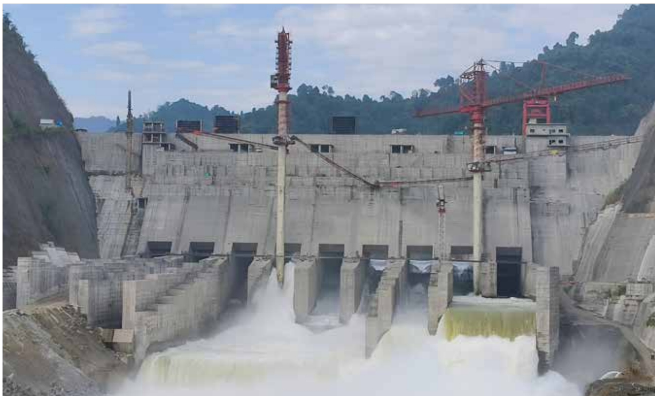
116 M HIGH CONCRETE GRAVITY DAM – 2000 MW SUBANSIRI LOWER (ARUNACHAL PRADESH)
