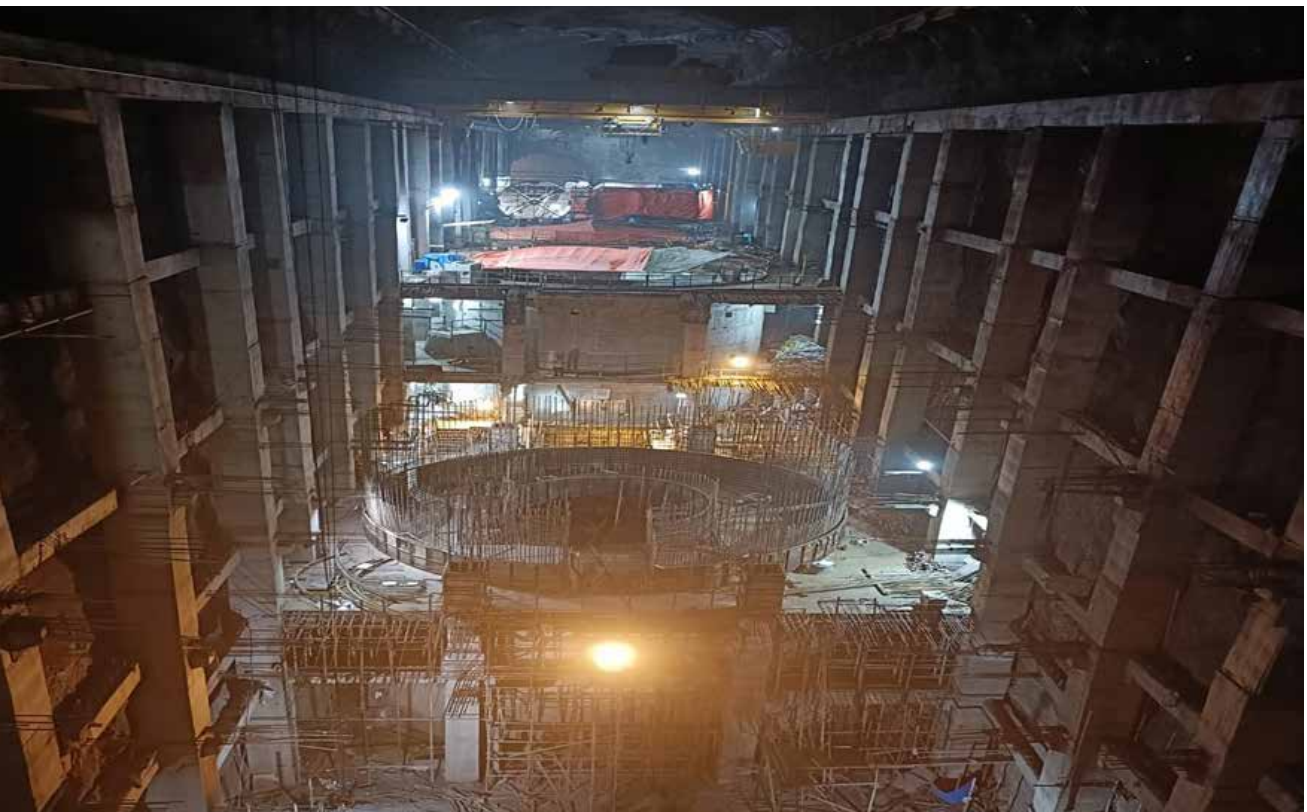
UNDERGROUND POWER HOUSE UNDER CONSTRUCTION – 500 MW TEESTA-VI (SIKKIM)
