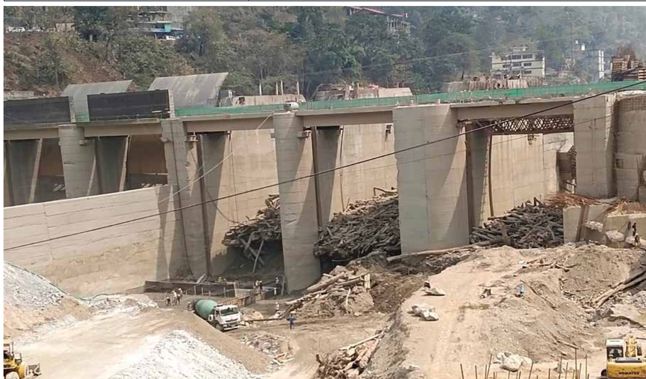
44 M HIGH CONCRETE GRAVITY DAM UNDER CONSTRUCTION – 120 MW RANGIT-IV (SIKKIM)
