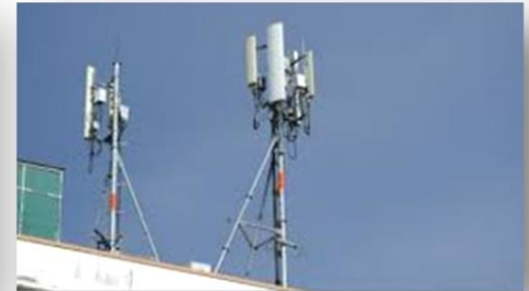
Roof Top Tower
