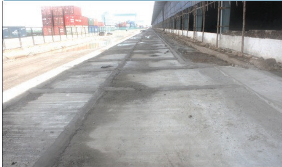
Road between Fertilizer Shed & RMGC Yard
