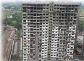
Finishing work in progress
