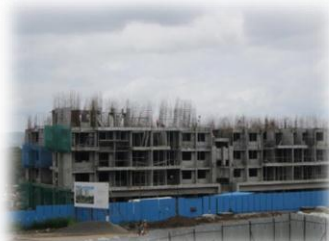
Slab for 3rd floor
