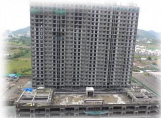
Finishing work in progress
