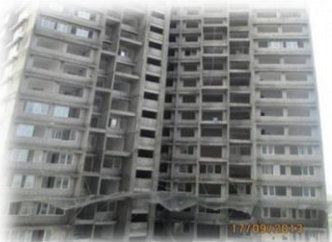
Aluform completed for 18 th floor
