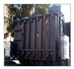
Kirloskar Electric Company Limited has successfully exported a Generator Duty transformer of 24 / 30 MVA, 115 / 38.5 / 10.5 kV for a hydro-electric project in Song-Giang, Vietnam through an EPC Contractor. The windings of the transformer are rated for full power of 30 MVA with any of the combination of the pair of windings and for the combined operation of all the windings with suitable loading distributed among the secondaries.
