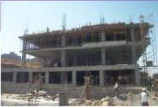
4th Slab in May 2013
