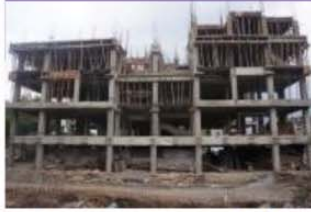
Site progress - June 2013
