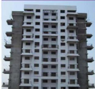
Site progress - April 2013
