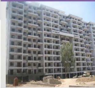
Flooring completed till 10th floor
