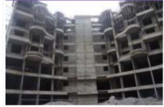
Site progress - June 2013
