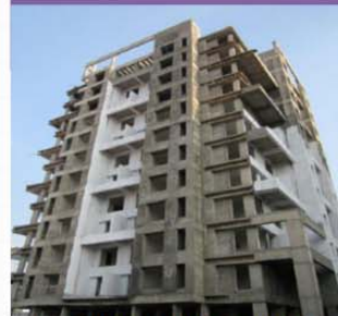
Plaster till 6th floor & tiling work till 4th floor completed
