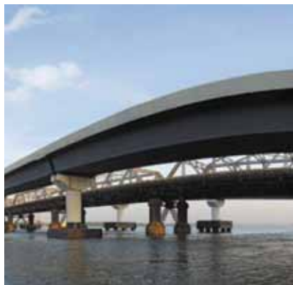
KASHELI BRIDGE MAHARASHTRA
