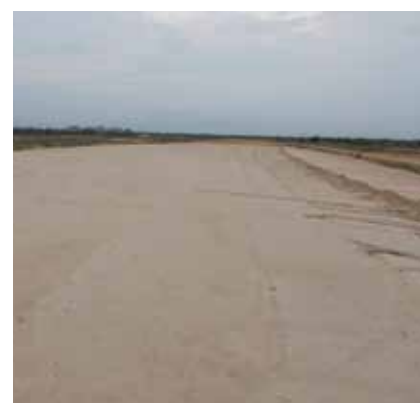
JAIPUR RING ROAD RAJASTHAN
