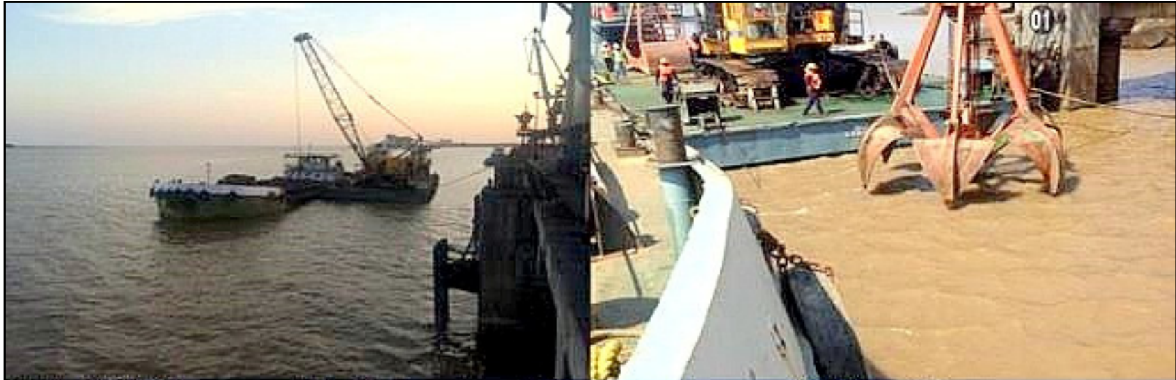
Dredging at berth and Channel
