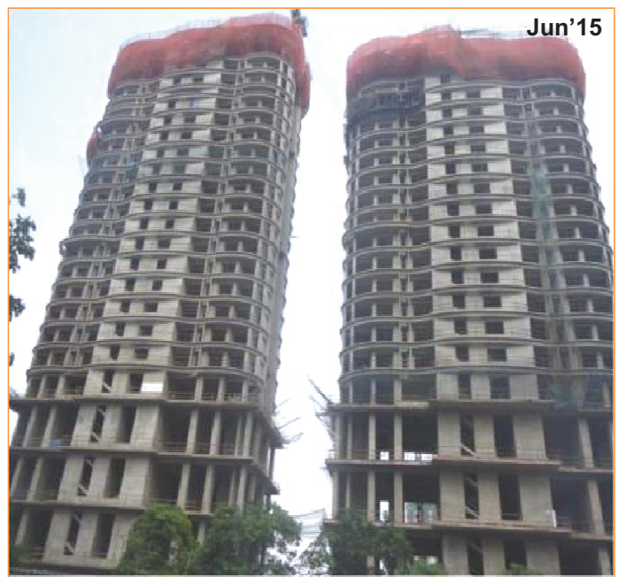
✓ Tower A & B - RCC work upto 24 th slab & upto 22 nd slab completed respectively
