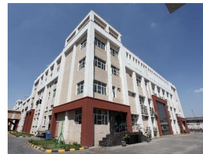
RFL 7A & B - Bahadurgarh
