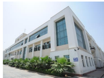
RFL 6A & B - Bahadurgarh
