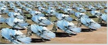
**Solar Thermal** - Uses parabolic disc technology to capture thermal energy basted on the solar thermal effect
