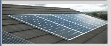
**Photovoltaic Solar Panels** - A typical silicon PV cell is a thin wafer consisting of phosphorous doped (Ntype) silicon on top of a thicker layer of borondoped (P- type) silicon. An electric field is created near the top surface of the cell where these two materials are in contact (the P-N junction). When sun light strikes the surface of PV cell, this electrical field results in a flow of current when the cell is connected to an electrical load.
