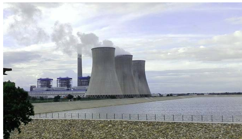
Talwandi Sabo 1980MW Power Plant
