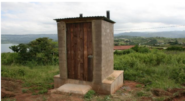
100 toilets in adopted village
