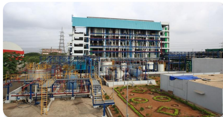
Agro Chemical Facility - Talaja
