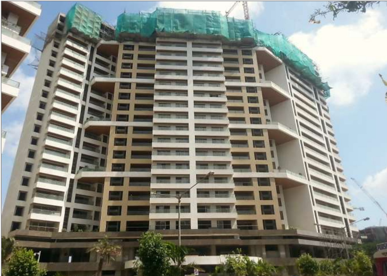
Final stage of RCC WIP & Finishing WIP
