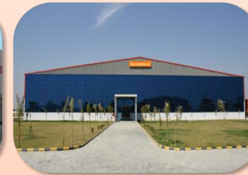
Unit 9 - Ahmedabad, Gujarat
