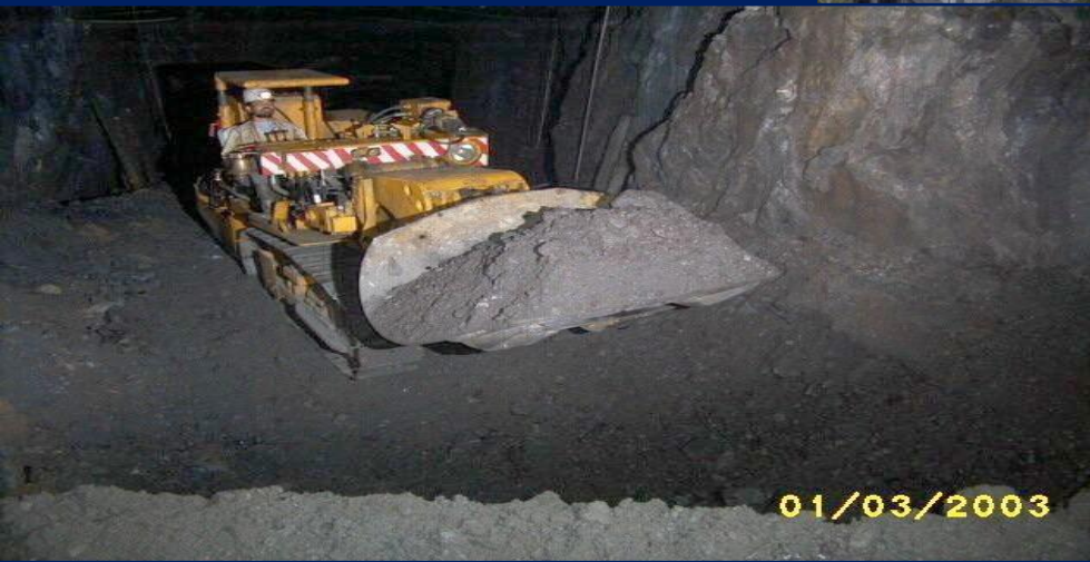
Production Shaft & Cable Bolting Operations
