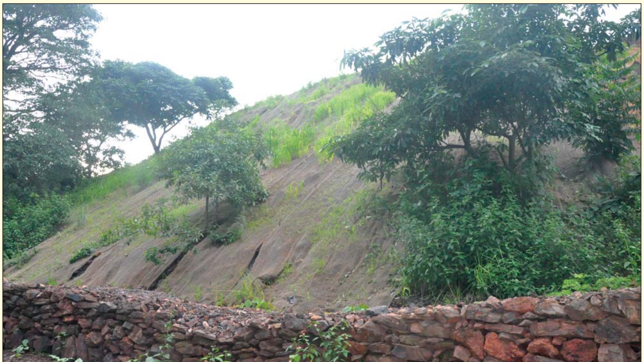
Coir Mat with Grass Seedling at SAIL's MIOM Waste Dump. The mines of Raw Materials Division tirelessly work to maintain the forest ecology and environment which is essential for scientific and sustainable mining.
