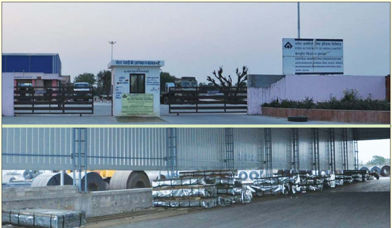
SAIL's modern Stock Yard at Jaipur - continuously focussing on developing fatigue free surrounding for proper storage and ease of handling materials thereby enhancing customer satisfaction.
