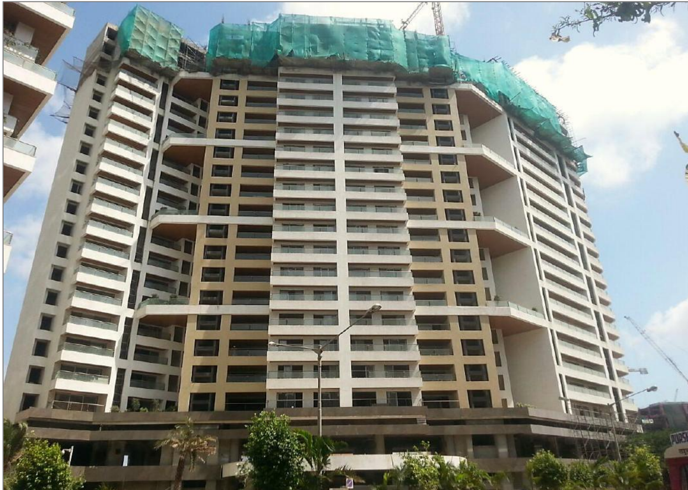
Final stage of RCC work-in-progress Finishing WIP
