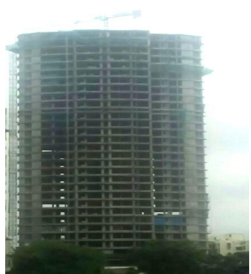
Terrace slab only remaining
