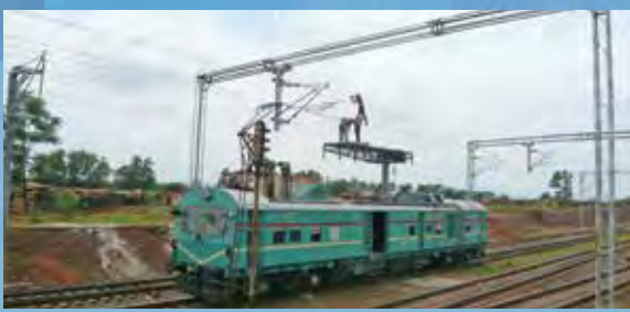
OHE job is in Progress.
