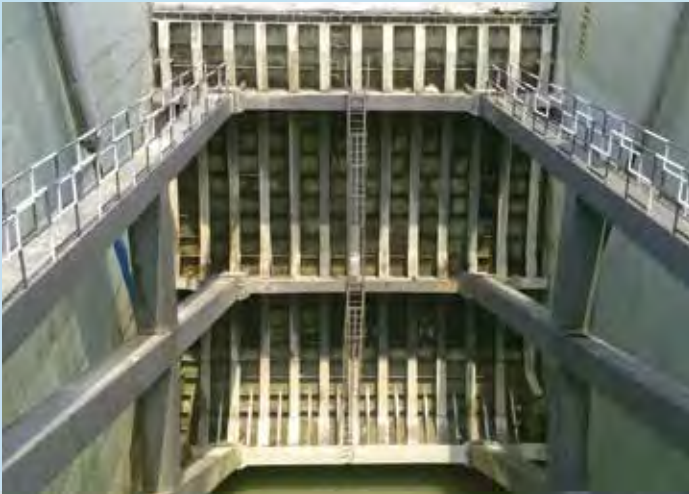
High Head (45 M) Top Seal Radial Gate erected at an elevation of 7216 ft., at Parbati Hydroelectric Project - Stage II (800 MW), Himachal Pradesh
