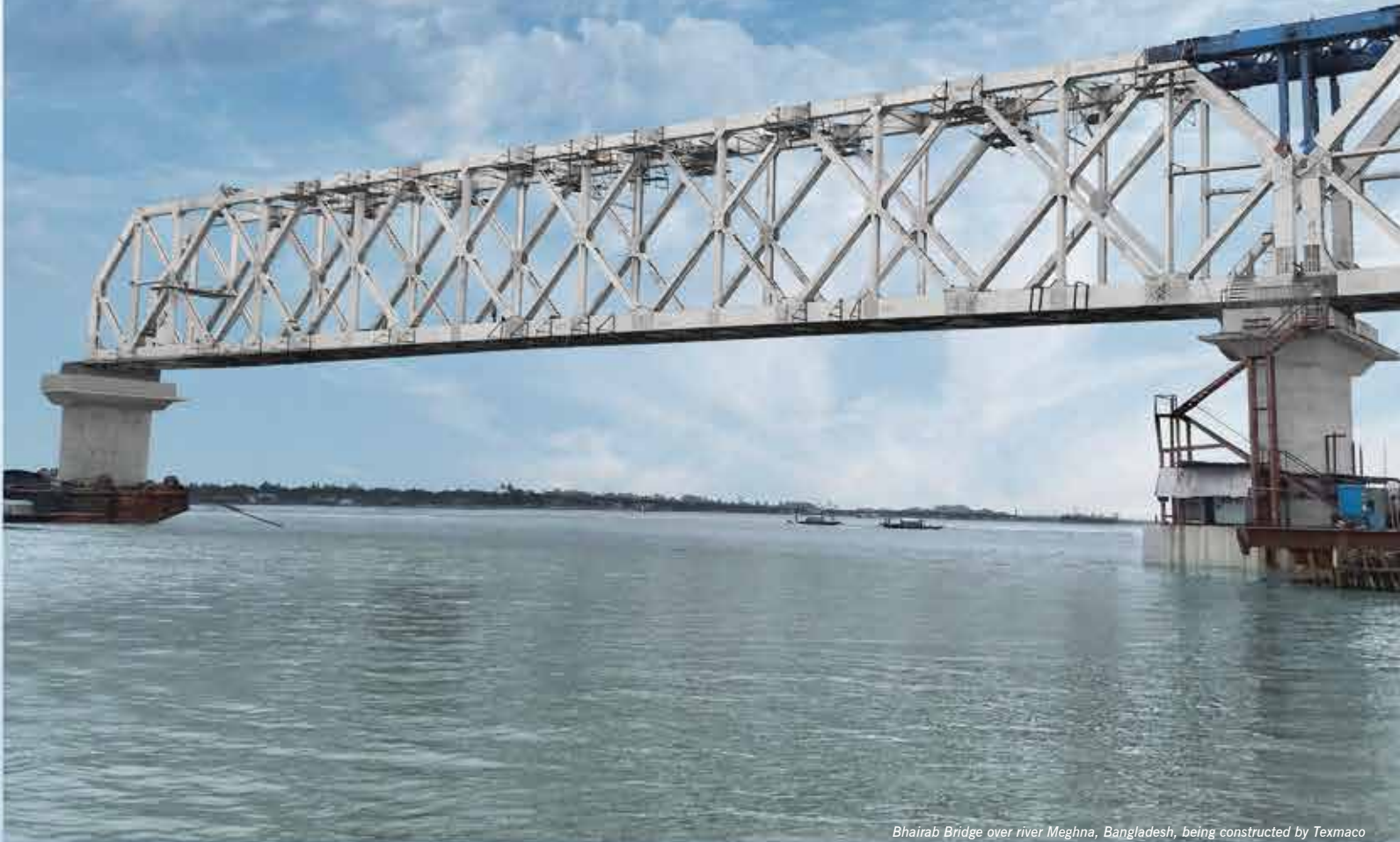
Bhairab Bridge over river Meghna, Bangladesh, being constructed by Texmaco
