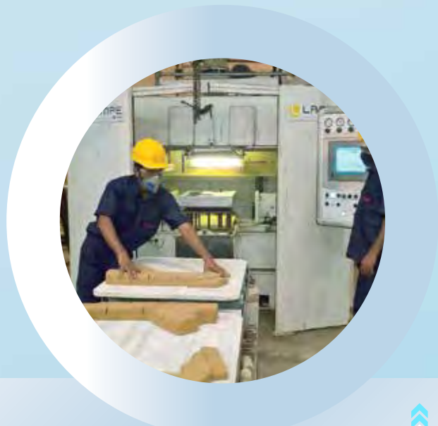
PLC controlled High Speed Core Shooter/ Blower from Laempe, Germany, installed at the Steel Foundry
