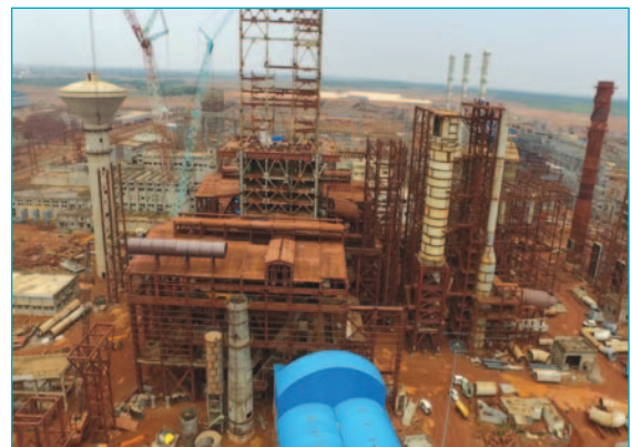
Overview of Blast Furnace at NISP, Nagarnar (under construction)
