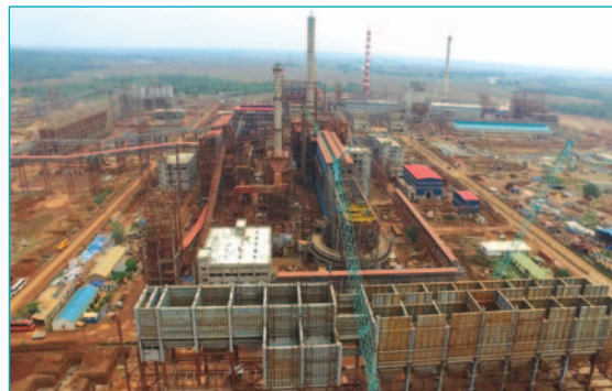
Overview of Sinter Plant at NISP, Nagarnar
