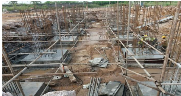
Captive power plant foundations
