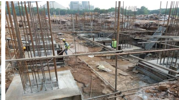
Captive power plant foundations
