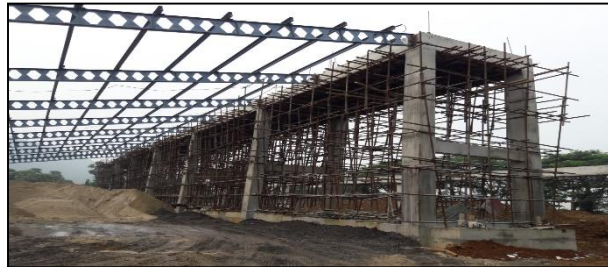
Raw Material storage facilities
