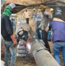
Thumbli Water Pipeline– Cairn Energy India – Rajasthan
