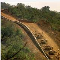
Panvel Dabhol Pipeline Project–Gail Ltd - Maharashtra
