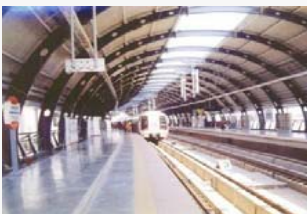
Elevated Metro Stations, DMRC, Delhi
