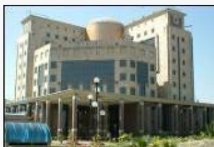
Power Grid Corpn., Gurgaon
