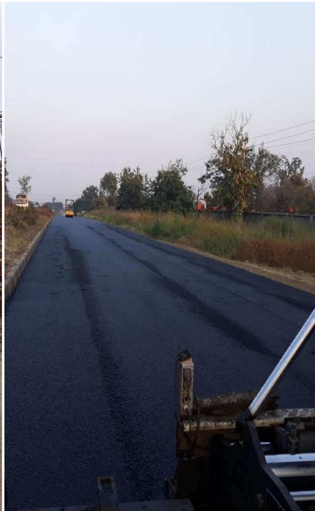
Major Maintenance Work at Nagpur-Kondhali Section of NH-6
