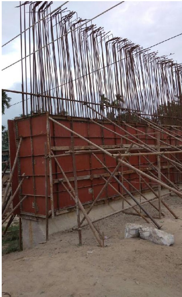
Vehicle Underpass at Moran Bypass of NH-37
