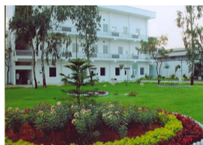
Jeedimetla, Telangana, India SUVEN R&D–Pilot Plant
