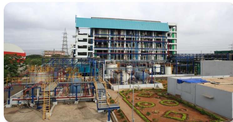
Agro Chemical Facility - Taloja
