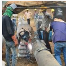
Thumbli Water Pipeline– Cairn Energy India – Rajasthan
