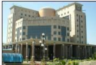
Power Grid Corpn., Gurgaon
