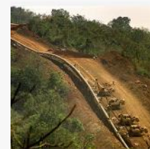
Panvel Dabhol Pipeline Project–Gail Ltd - Maharashtra
