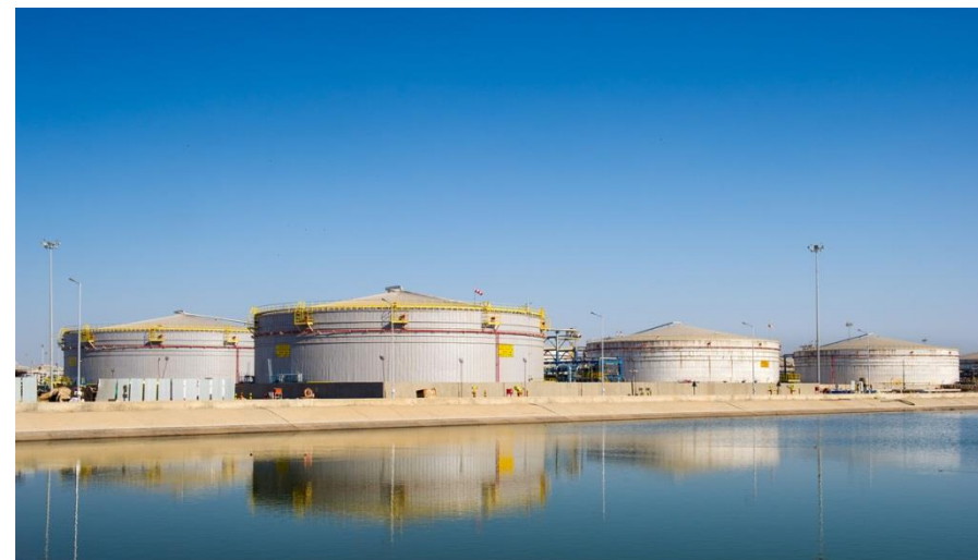
Rajasthan: Mangala Processing Terminal
