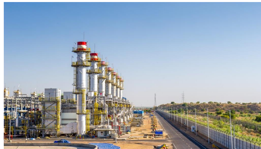
Rajasthan: Steam Turbine Generators at Mangala
