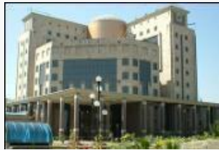
Power Grid Corpn., Gurgaon
