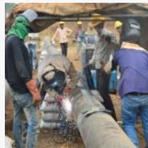
Thumbli Water Pipeline– Cairn Energy India – Rajasthan
