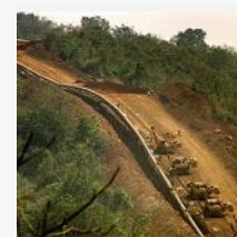
Panvel Dabhol Pipeline Project–Gail Ltd - Maharashtra
