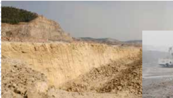
Side-Cast Blast in 55 mtr dragline bench with pre-splitting in Sasan Power Limited (Reliance), Singrauli giving reduction in material handling of dragline by over 40% by throwing blasted muck to de-coaled area
