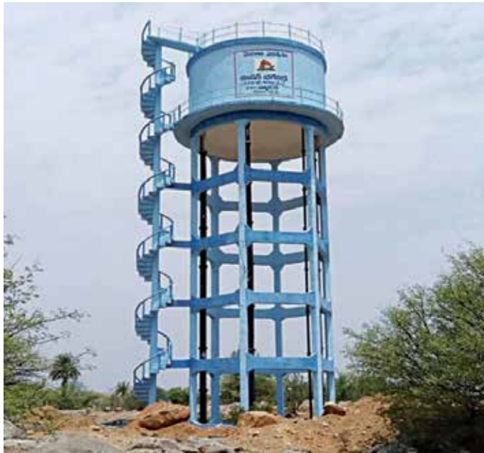
90 KL x 15 Mtr staging OHBR at Maldakal for Jurala (TDWSP) Project, in Telangana
