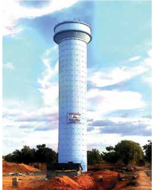
90 KL x 30 Mtr staging OHBR at Mallamdoddi for Jurala (TDWSP) Project, in Telangana
