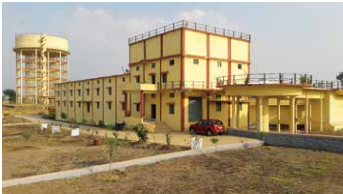
26 MLD capacity Water Treatment Plant at Chalisgaon City Water Supply Scheme, in Maharashtra
