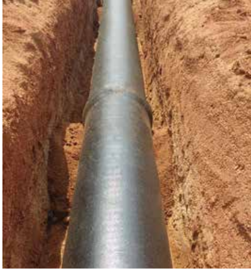
1000 mm dia DI K-7 pipeline at Jurala Segment for Jurala (TDWSP) Project, in Telangana
