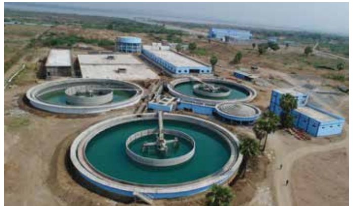
160 MLD Water Treatment Plant at Murmur Village Yellampally for Karimnagar (TDWSP) Project, in Telangana.
