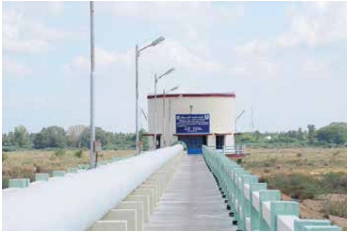
23 MLD capacity collector well at Pudukottai project in Tamilnadu
