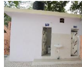
Toilet Facility Provided in PHC of Banipur
