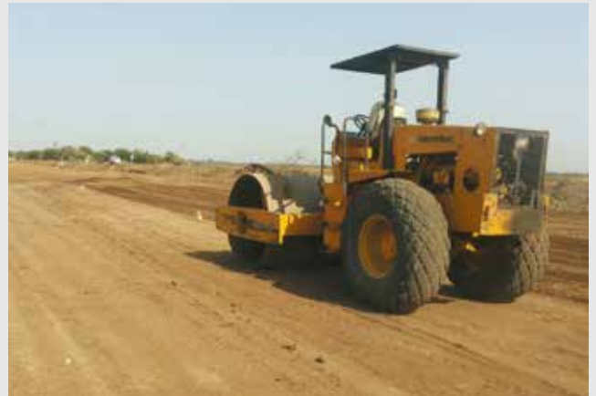
Work in progress on embankment top layer
