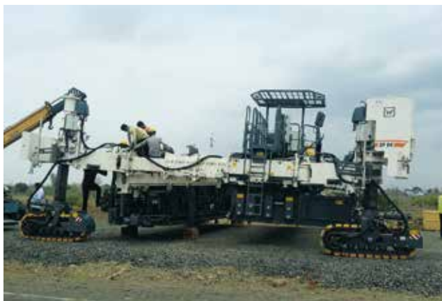
Wirtgen Slipform Paver used for pavement quality concrete
