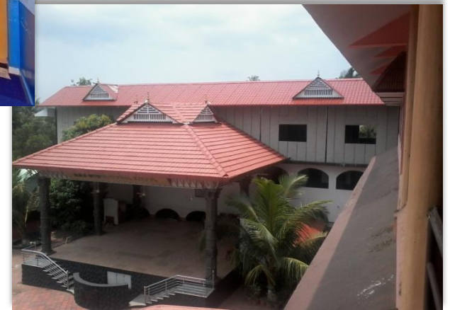
Roof Top Extension - (V-Panel )
