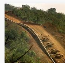
Panvel Dabhol Pipeline Project–Gail Ltd - Maharashtra
