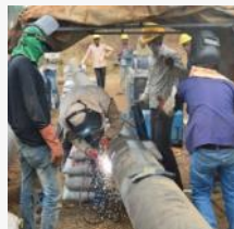
Thumbli Water Pipeline– Cairn Energy India – Rajasthan
