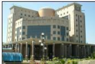
Power Grid Corpn., Gurgaon
