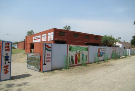
Renovation of Govt. Middle School
