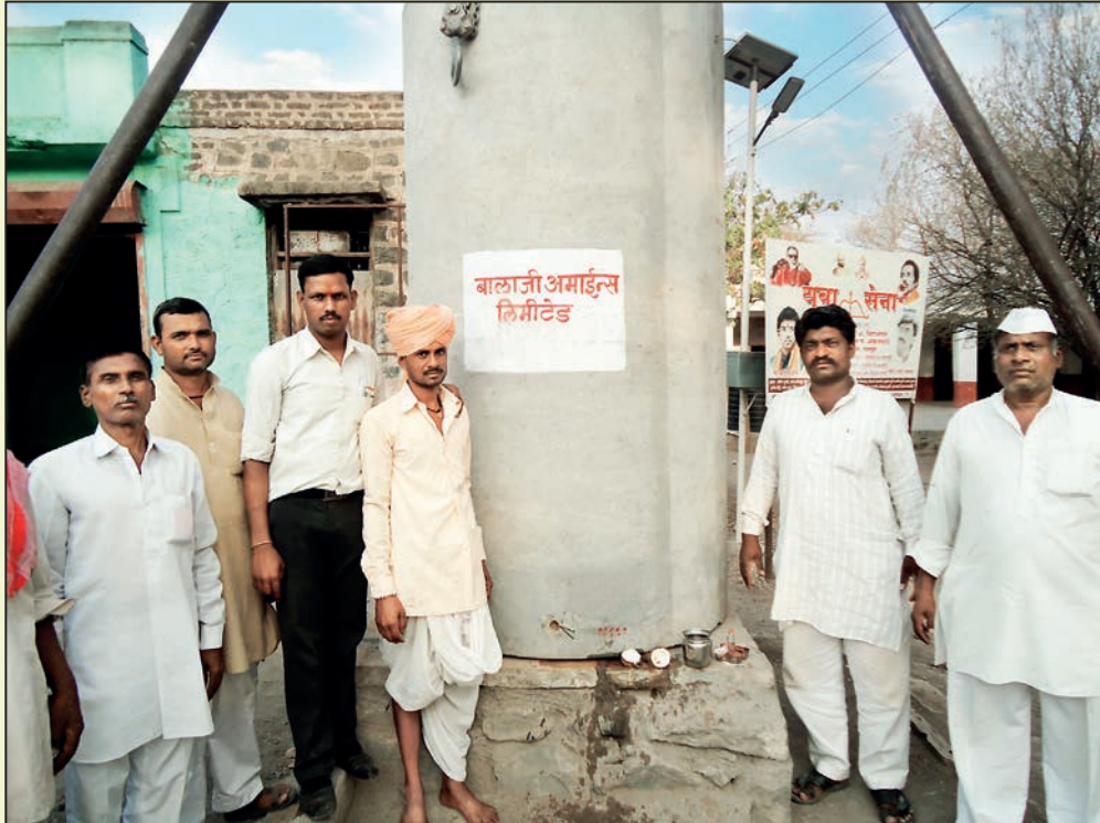
Distribution Water Storage Tank at Yetnal Village, Solapur District.
