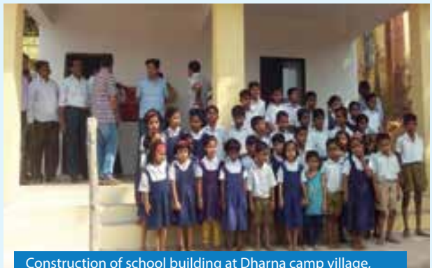
Construction of school building at Dharna camp village, Talaja, India
