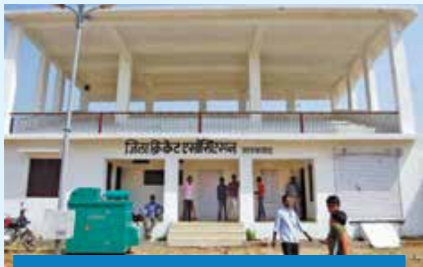
Construction of outdoor stadium at Jehanabad, Bihar, India
