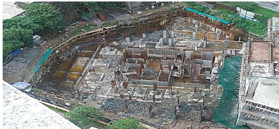
Tower B: Footing and rafting in progress
